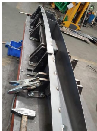
Figure 6. Welding tool in a real environment
