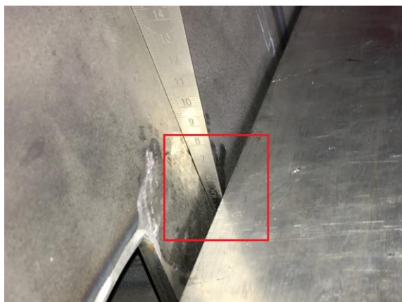
Figure 7. Pillar welding out of tool
